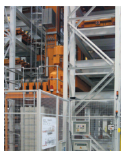
A high-bay crane at the Emden factory
